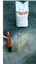
**Use granular absorbents if booms alone cannot absorb spill and dispose in Waste Bag in Spill Kit**
